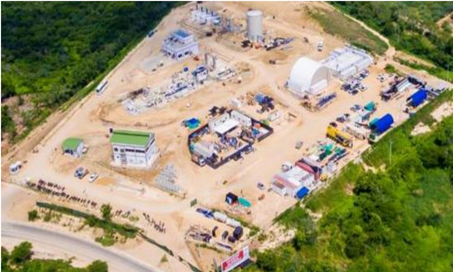
Progress SPEC. Construction On Shore - August 2016
