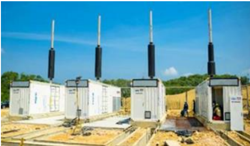
Installation of chimneys and generators - August 2016
