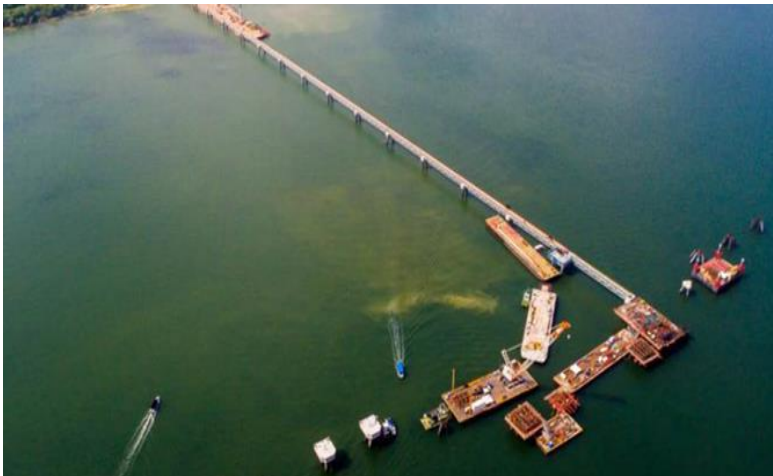
Construction Off Shore - August 2016
