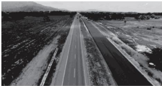
Picture 1. Ruta del Sol PR 51+000 south carriageway
