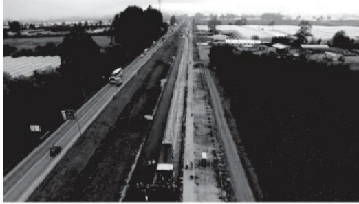
Picture 2. CCFC dual carriageway PK 18+850
